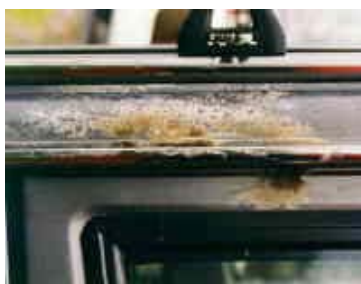
Close-up of roof strike
